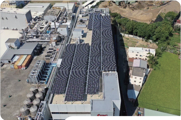
▼ Phase 2 solar panels
